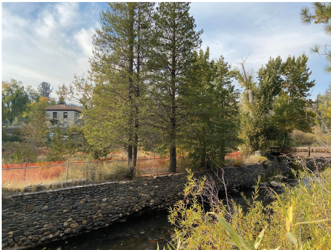
Photo 1. Existing conditions along Markleeville Creek with rock floodwall shown isolating the floodplain (October 13, 2023).
