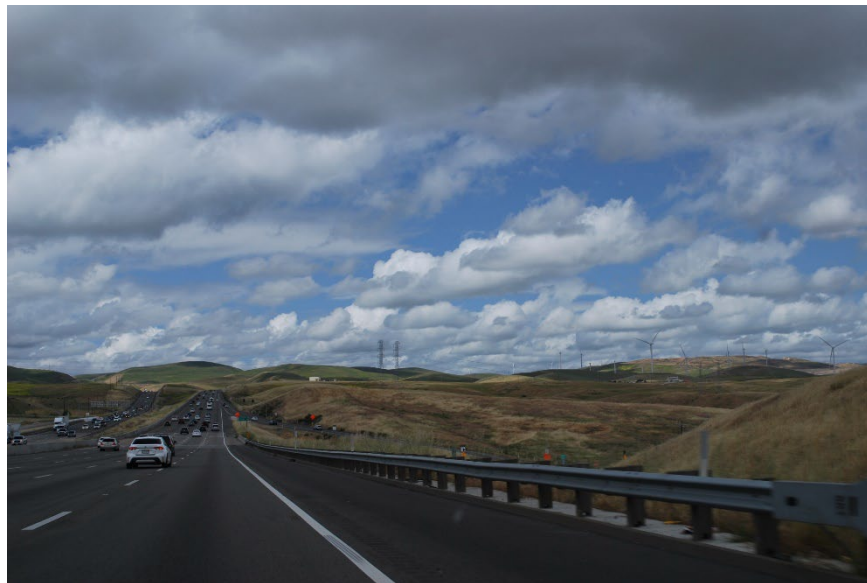
Figure A3.2-19: Key View 10 (I-580 Westbound at Grant Line) - Existing
