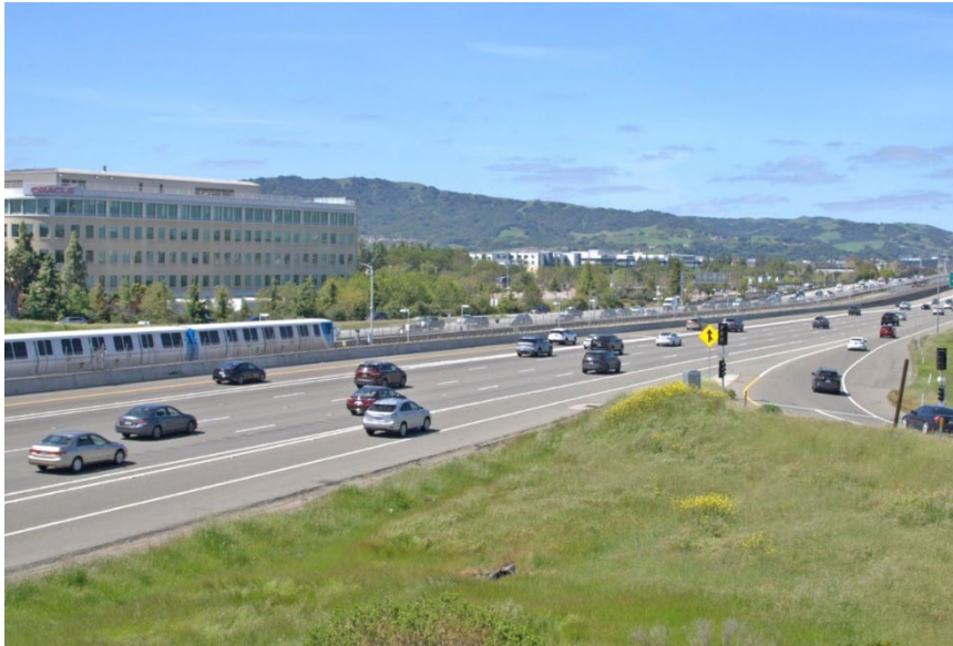
Figure A3.2-5: Key View 3 (Hacienda Drive) - Existing
