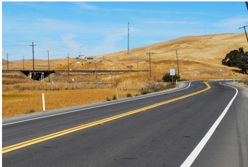
Figure A3.2-11: Key View 6 (Altamont at Dyer Road) - Existing
