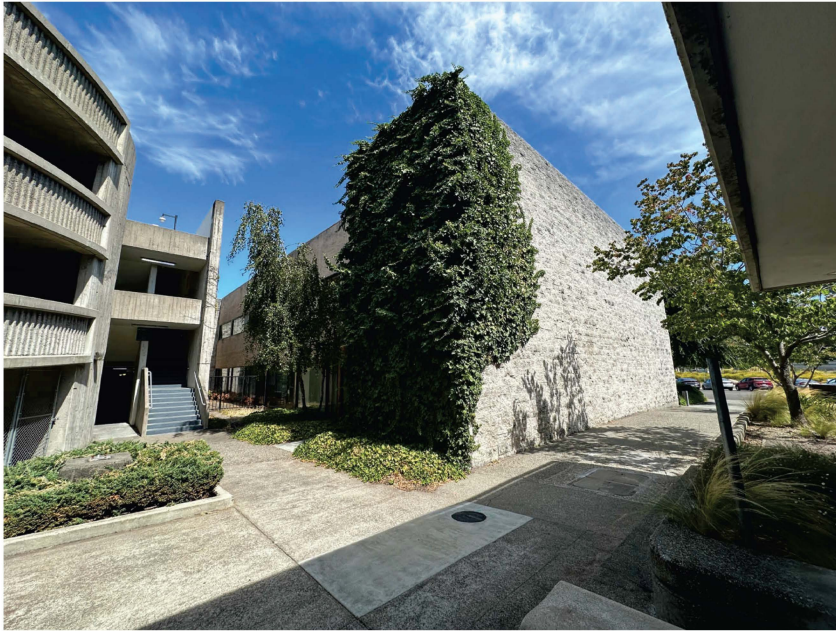
Photo A: View of northwest corner of Chamber Building facing southeast.
