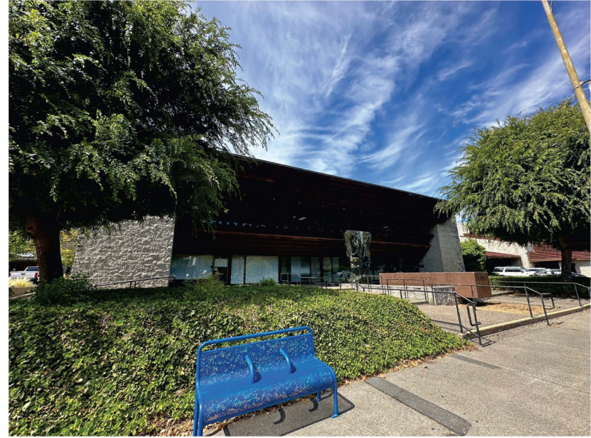
Photo B: View of Chamber Building from 1st Street facing north.
