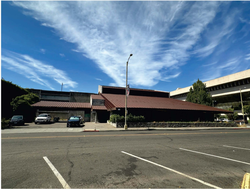
Photo A: View of old bank building from 1st Street facing north.
