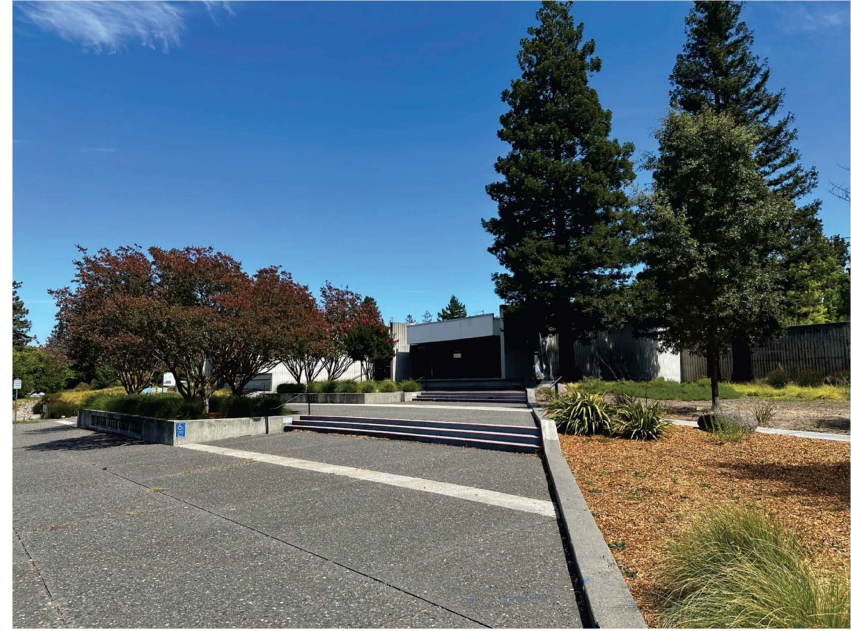
Photo F: View of northwest corner of City Hall facing southeast.
