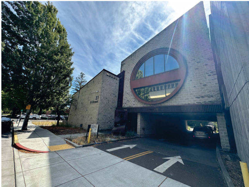
Photo C: View of old bank building from D Street facing west.
