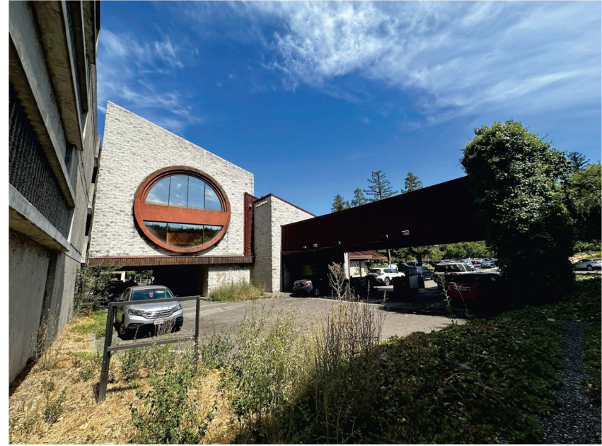
Photo B: View of west corner of old bank building facing east.
