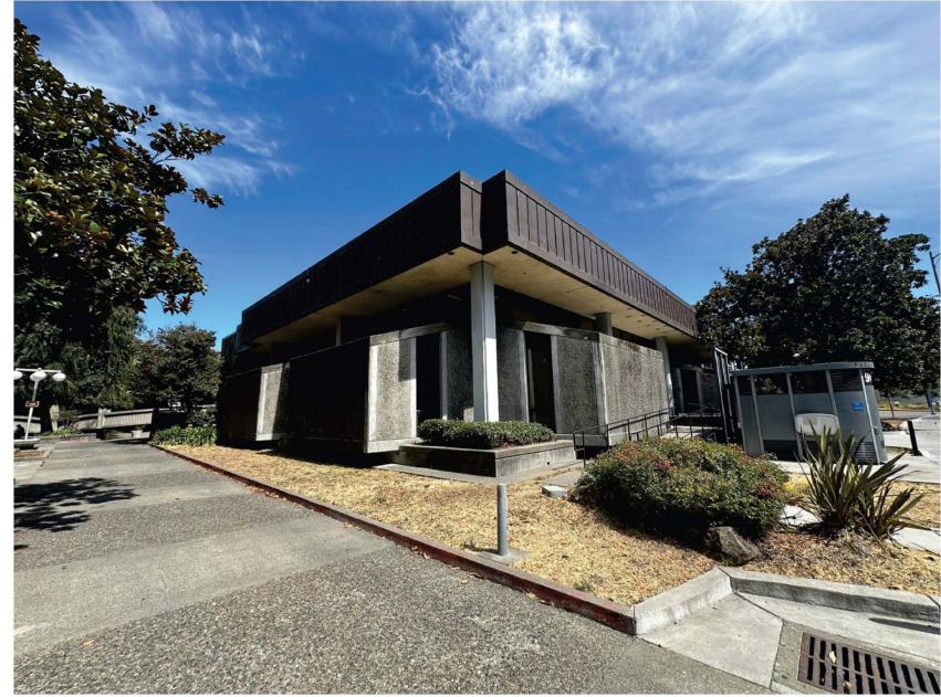
Photo B: Northwest Corner of Annex facing southeast.
