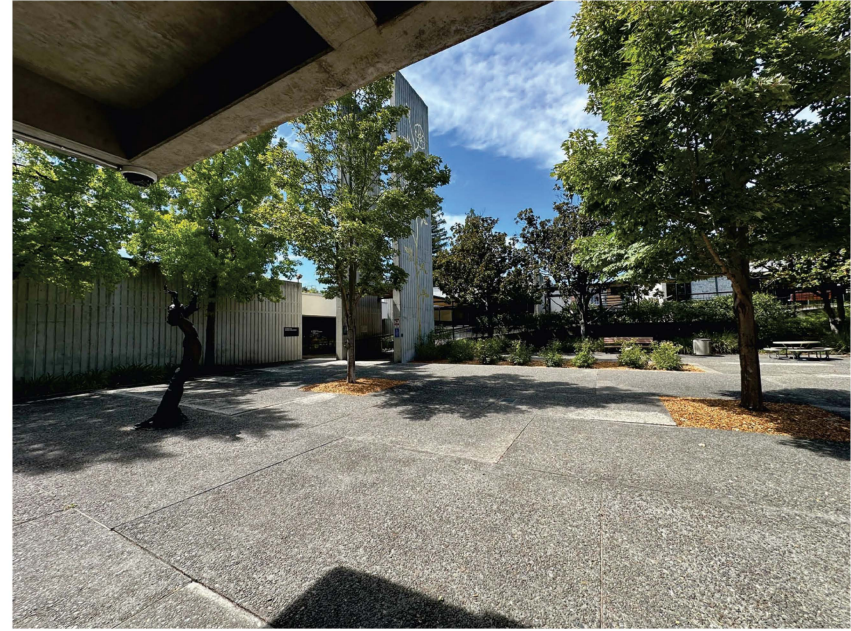
Photo B: View of Center of plaza facing northwest.
