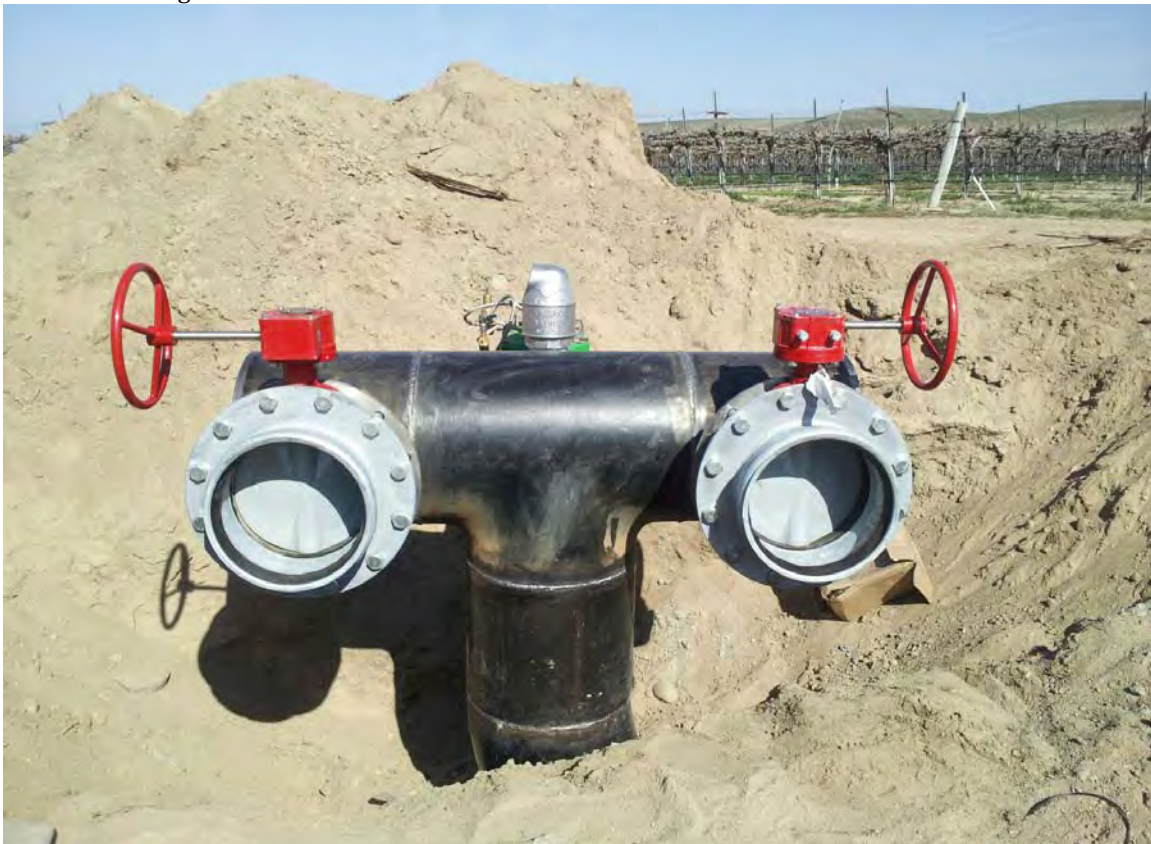
Photo 10. Representative photo of how waterline with valves will “daylight” outside top of bank of drainages. Flexible HDPE pipe will be attached and then run overland at drainage crossings.
