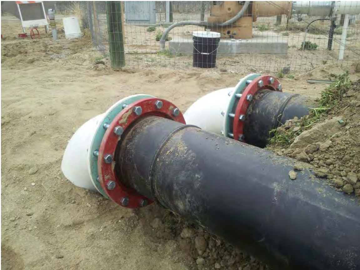
Photo 11. Representative photo illustrating connection of HDPE pipe and underground pipe.
