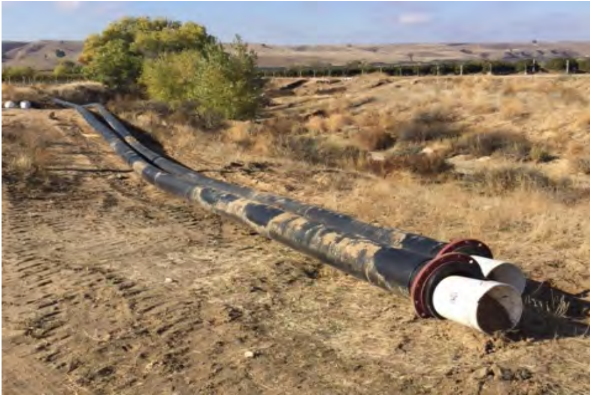
Photo 9. Representative photo from another site showing the flexible HDPE pipe to be laid above ground over the drainage features.
