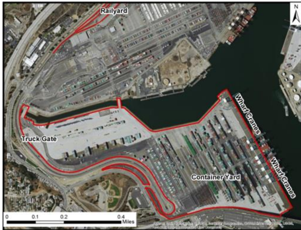
16 Figure ES-1: Berths 97-109 (China Shipping) Container Terminal
