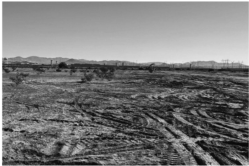
Photo 5 - Recently disturbed area on the project site.
