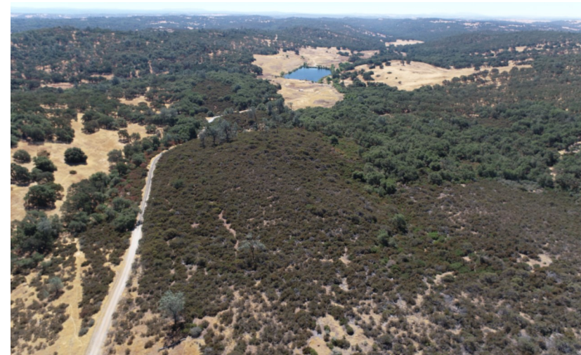
Photo 20. Project Overview – Quarry Pond in the Background, Facing South 16 Aug 2024
