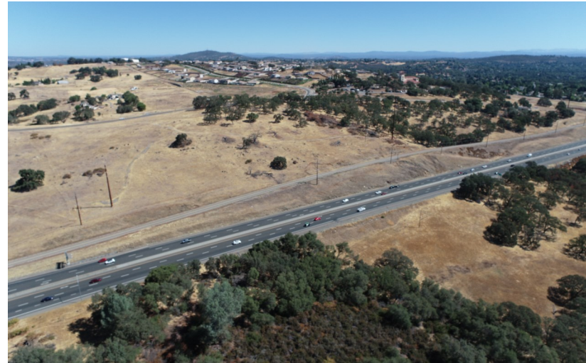
Photo 22. Offsite Infrastructure – Dry Utilities Extension, Facing Northeast 16 Aug 2024
