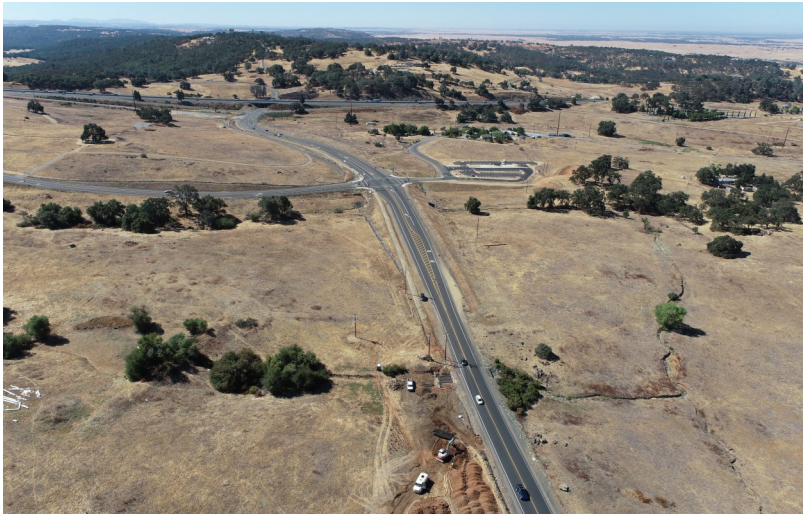
Photo 21. Offsite Infrastructure – Bass Lake Road Interchange, Facing South 16 Aug 2024
