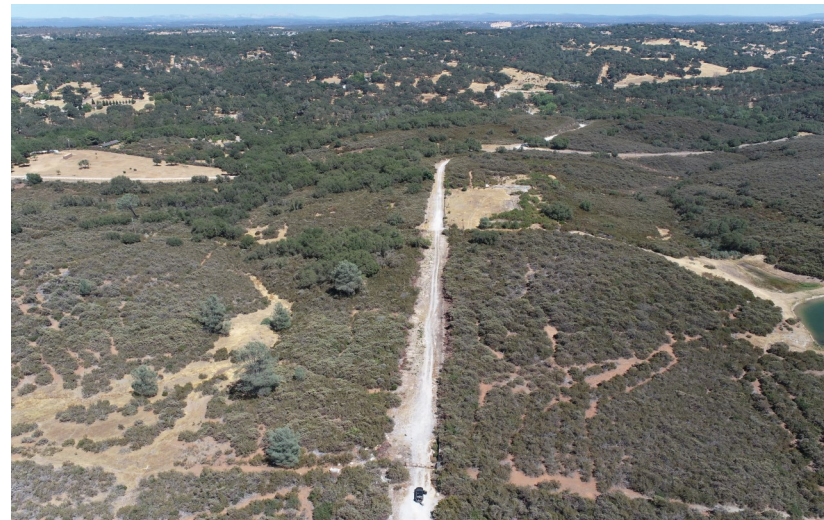
Photo 24. Offsite Infrastructure – Sewer Line, Facing East 16 Aug 2024
