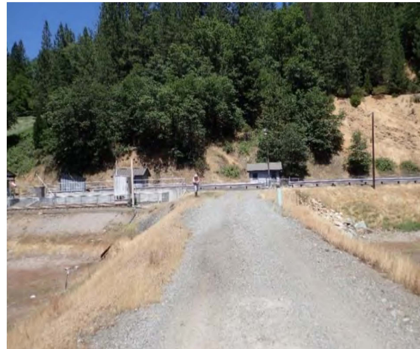
Photo 4.4-3. Bank between Percolation Pond 3 and 4 (Pond 4 on the right)
