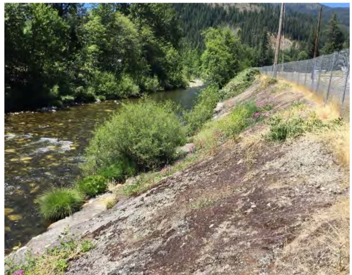
Photo 4.4-1. Sacramento River at new outfall location, facing
