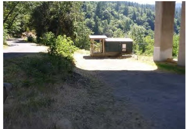
Photo 4.1-4. I-5 Lift Station, facing east from under the I-5 overpass.
