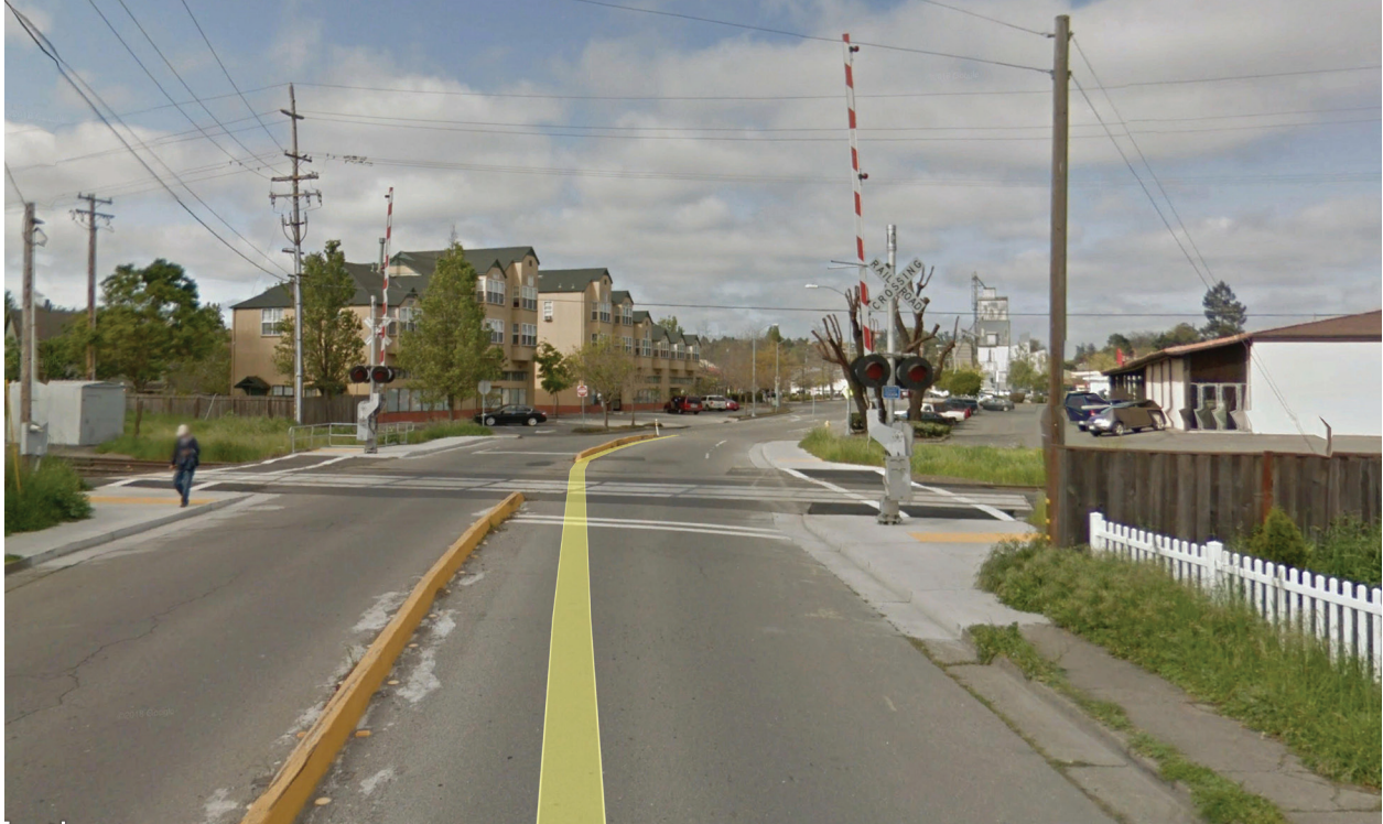
Prior Payran Street Crossing Improvements, at the time of publication of Draft EIR
