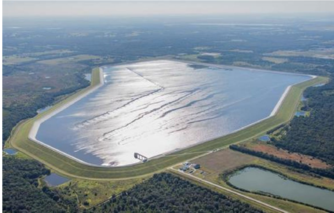
C.W. Bill Young Reservoir, Tampa Bay Water (FL) Flow Rate: 0.08 scfm/ft
