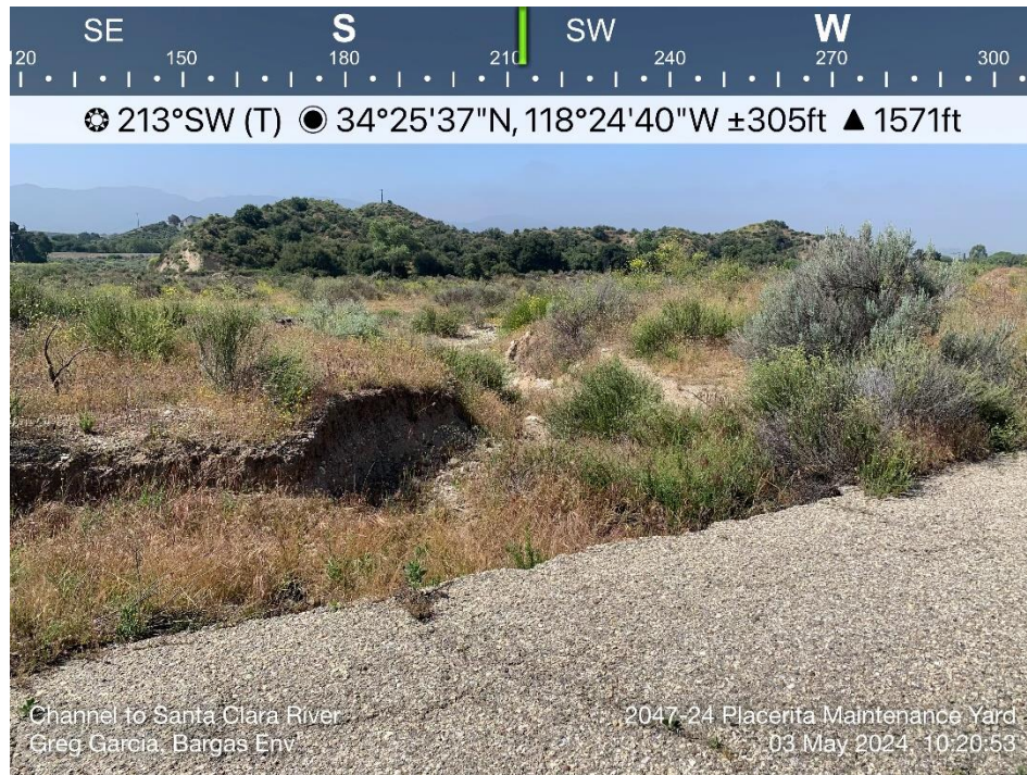
Picture 7: Erosional undercutting on Norland Drive.
