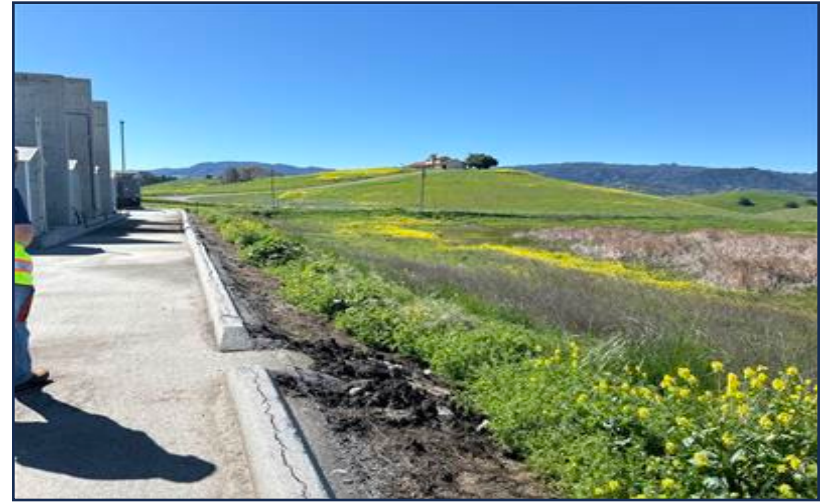
Photo 3b. View of seasonal wetland and facility pad curb. Photo taken facing 317 NW on 3/24/2025.
