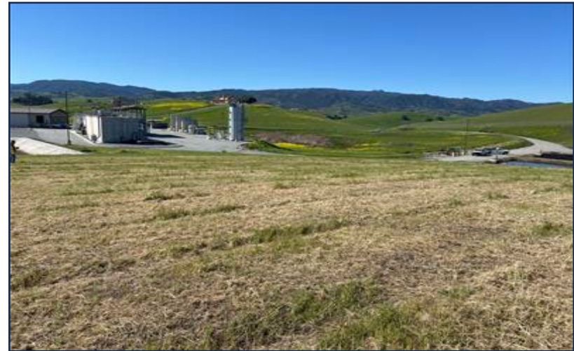
Photo 5a. Photo of the drying bed and facility from the mowed grassland east of the drying bed, Photo taken facing 180 degrees S on 3/24/2025.
