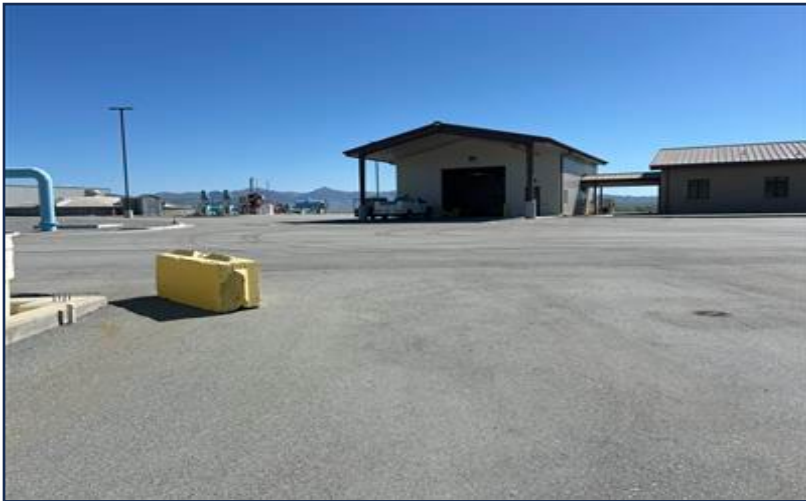
Photo 2a. View of the paved facility area where the new chemical storage tank will be placed. Photo taken facing 240 degrees on 3/24/2025.
