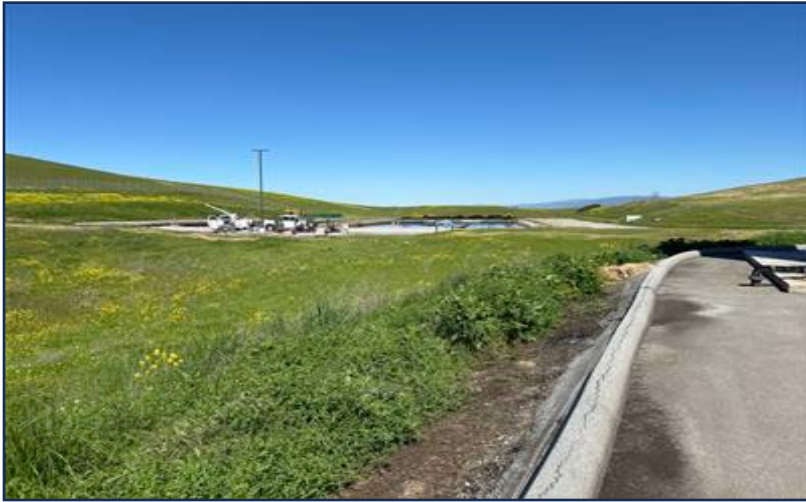
Photo 3a. View of the drying beds from the main facility pad. Photo taken facing 181 degrees S on 3/24/2025.
