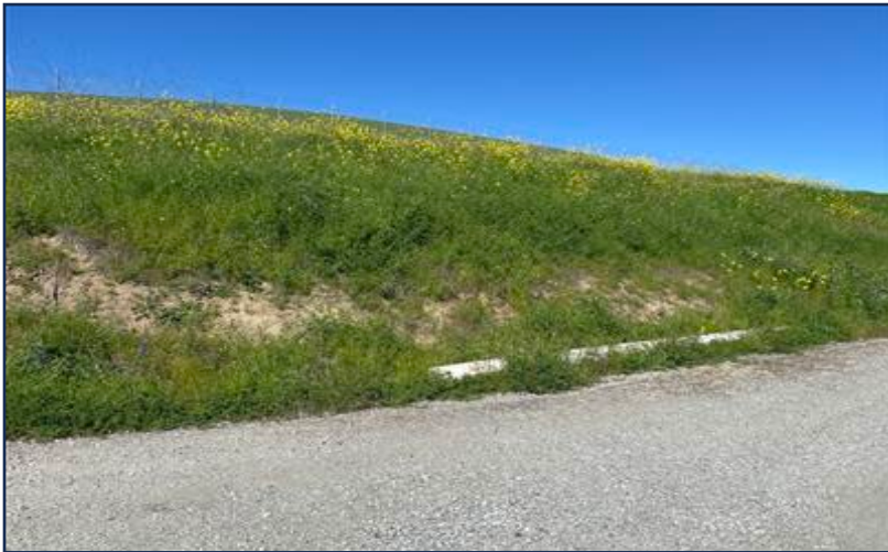
Photo 9b. View of the slope along the exit road. Photo taken facing 274 degrees west on 3/24/2025.
