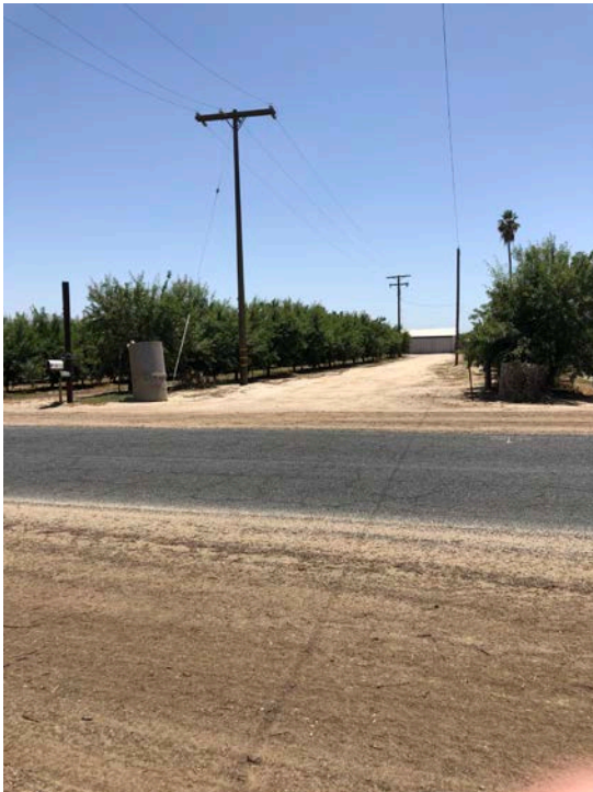
Photo 1: Infrastructure along northern boundary of project site. Source: 4-Creeks, Inc. 5/31/18
