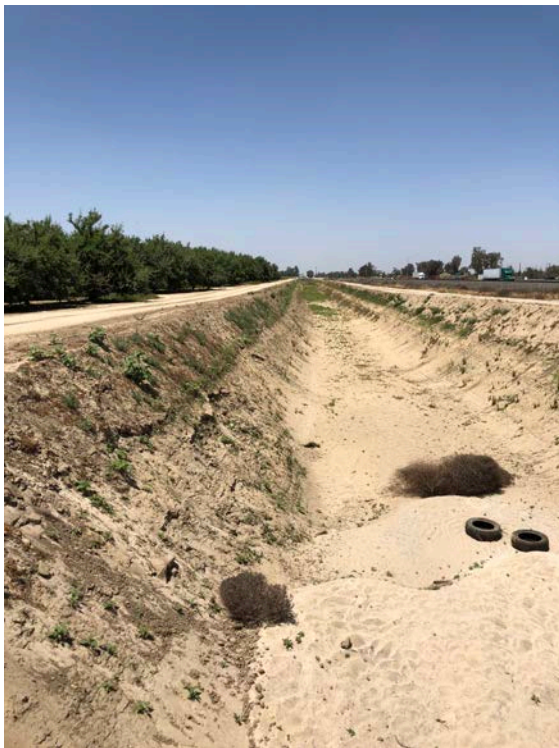
Photo 1: Canal running along eastern portion of project site. Source: 4-Creeks, Inc. 5/31/18
