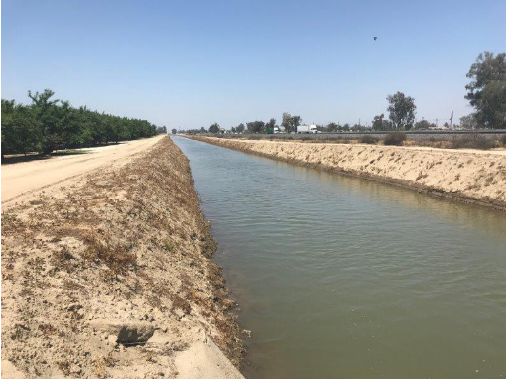
Photo 7 (above): Unnamed PID irrigation canal, two small segments of which pass through the project site along its eastern boundary.
