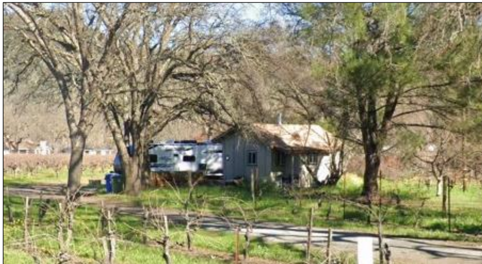
Figure 3: Subject Structure and Property Site. View from Grant Street. Source: Google Maps, 2024.
