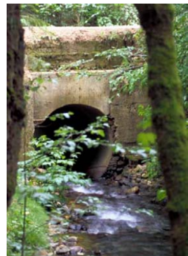
Figure 16: Culvert under rural paved road in the Sierra Nevada
