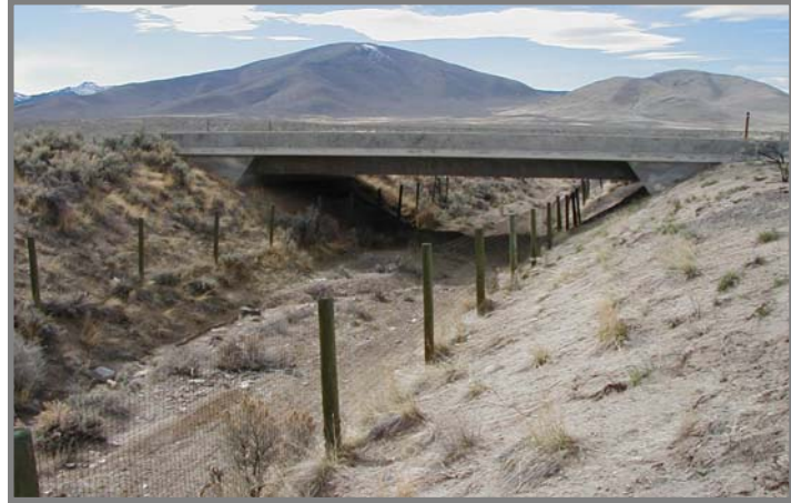
Figure 21: Wildlife Underpass, Sierra County. Photo courtesy Brian Ehler, Calif. DF&G
