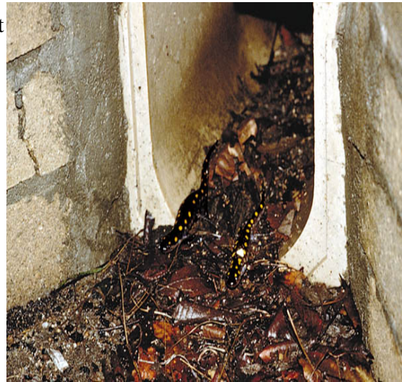
Figure 20: Salamanders exiting culvert. Photo: FHWA Critter Crossings website
