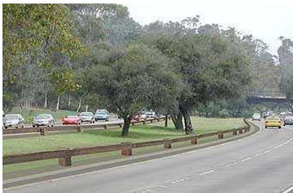
Figure 29: State Hwy. 163 median barrier.
