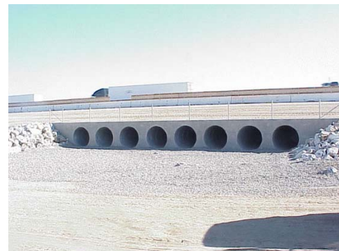
Figure 28: Culverts under I-15, San Bernardino County (Caltrans photo)
