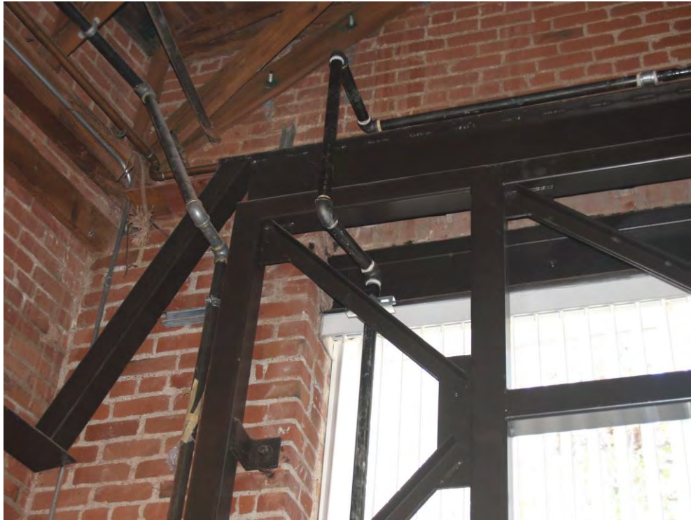
Internal structural reinforcement at façade.
