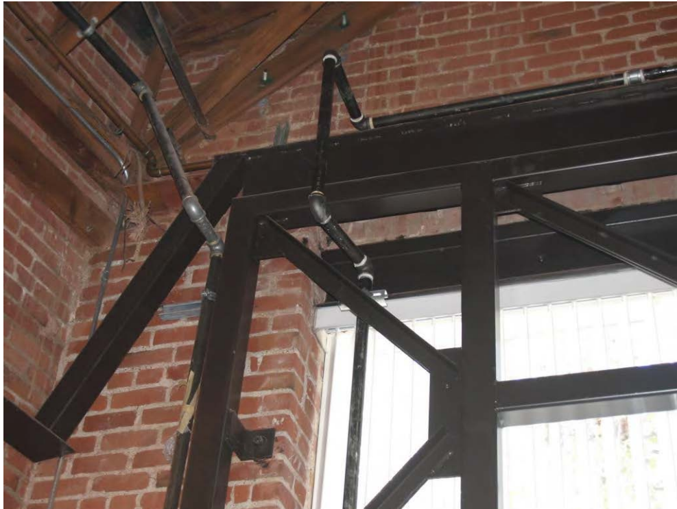
Internal structural reinforcement at façade.
