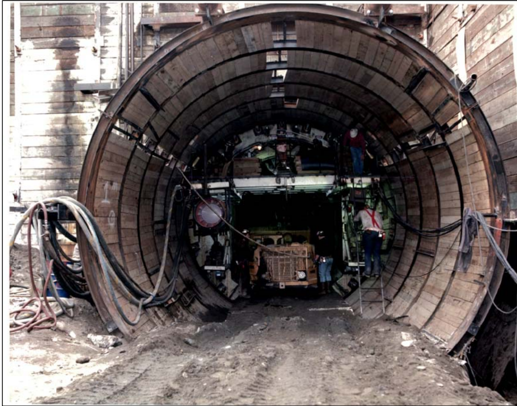
Photo No. 1. False tunnel sets at the South Tunnel Portal of YR Tunnel (south of LAUS) with tunnel shield and mucking machine in the background. Photo taken: 01/30/90. Source: SCRTD, 1990a.
