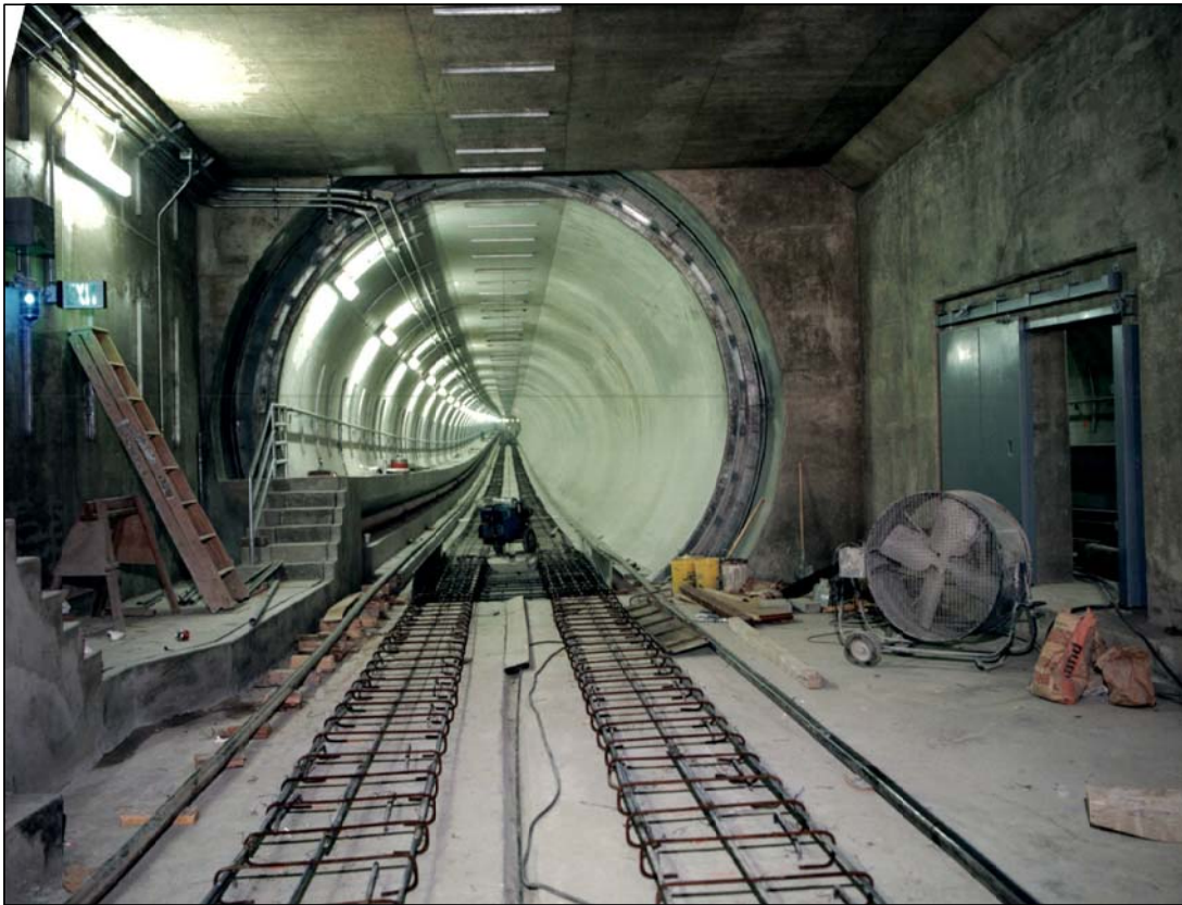
Photo No. 6. Interface between the box structure (LAUS area) on the YL side at Sta. 89+7 and the YL Tunnel (south of LAUS). Photo taken: 03/04/90. Source: SCRTD, 1990a.
