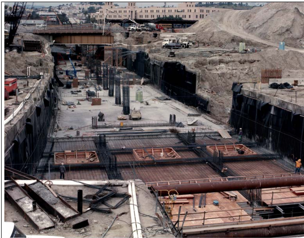
Photo No. 3. Mezzanine floor slab in place with column reinforcement steel protruding. The reinforcement for lift No. 4 of mezzanine floor is being placed in the foreground. Photo Taken: 01/30/90. Source: SCRTD, 1990a.
